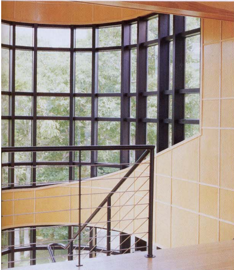
(left top and bottom) Vistawall aluminum frames and custom glass let in an abundance of natural light in the entranceway stairs. (below) The captain's wheelhouse wraps around the space.
